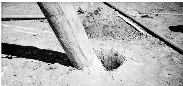
Erecting pole directly into ground, 1941
