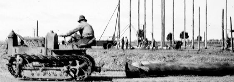
Moving and erecting poles for The Stick Shed, 1941
